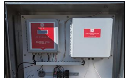
Installation of new 4-Gas Meter
