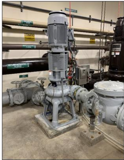
New drain pump No. 1
