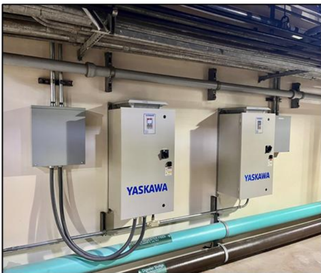
Installation of new process waste VFD's
