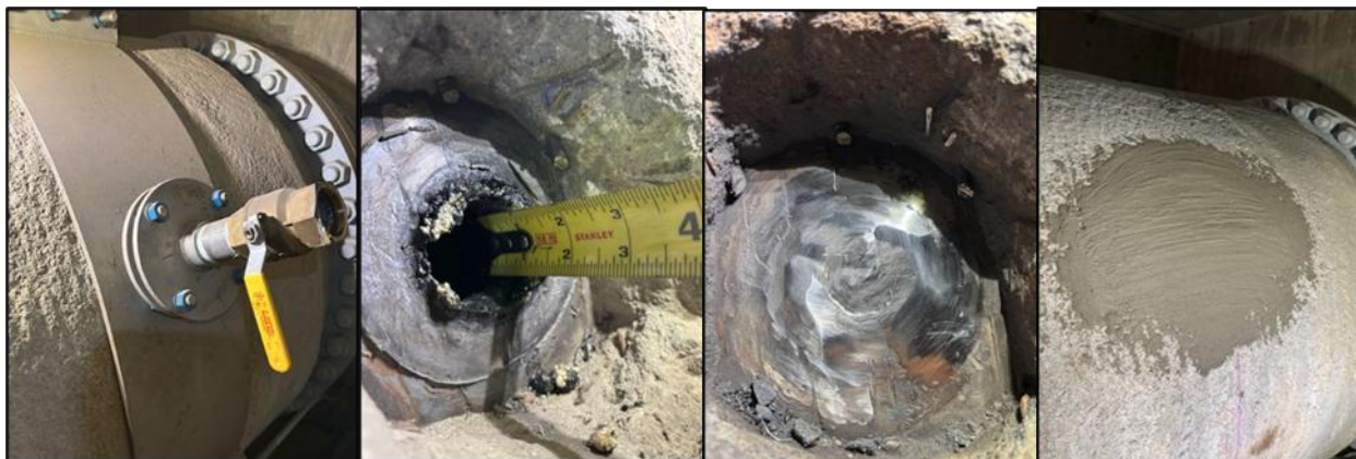
Removal of old unused flow meter, flowmeter insert welded over, and final concrete patchwork
