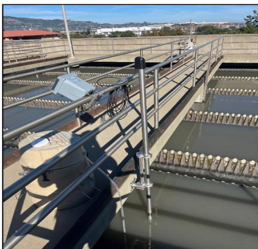
TSS probe installed in primary effluent
