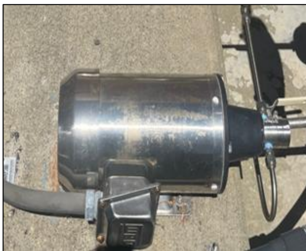
Two newly rebuilt hydrogen peroxide pumps for odor control
