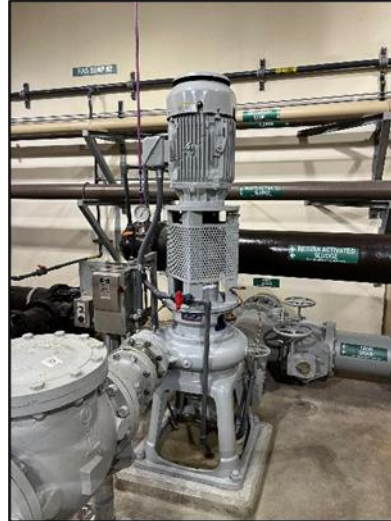
New drain pump No. 2
