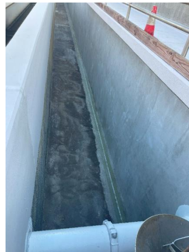
Fully rehabilitated Chlorine Contact Tank (CCT) No. 4 walls
