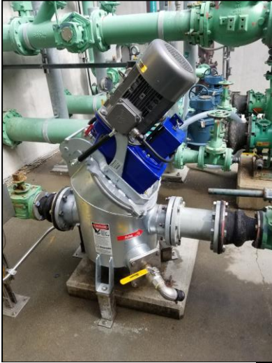
New grinder housing and motor
