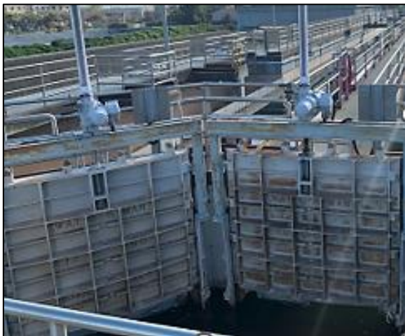
Before: cast iron gate and actuator
