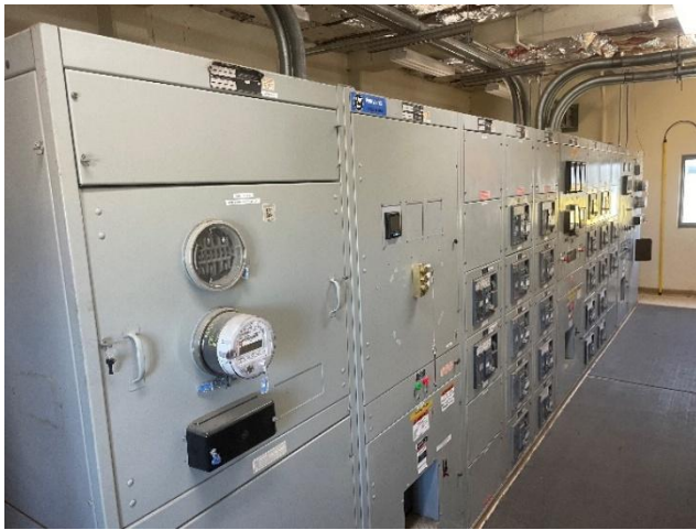
Main switchgear.
