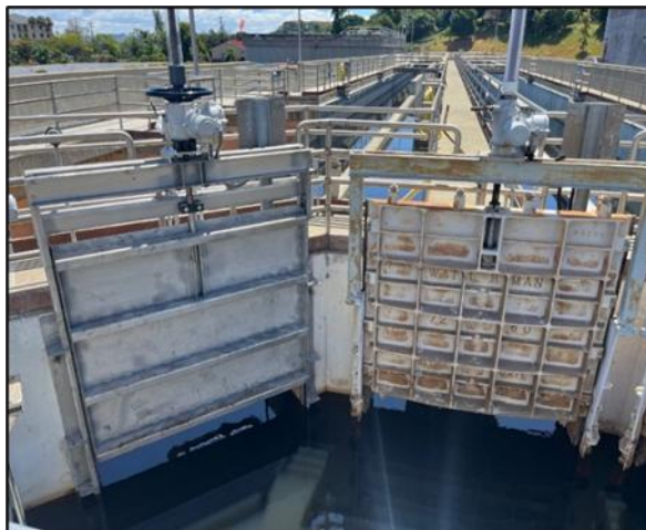
After: stainless steel gate and actuator
