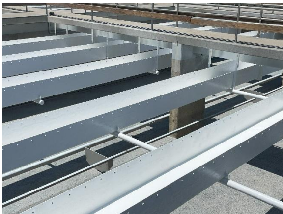
Recoated steel launder mechanisms on Primary Clarifiers
